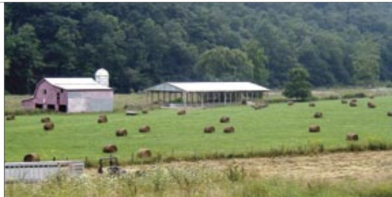
Roofed feeding area and manure storage facility.
