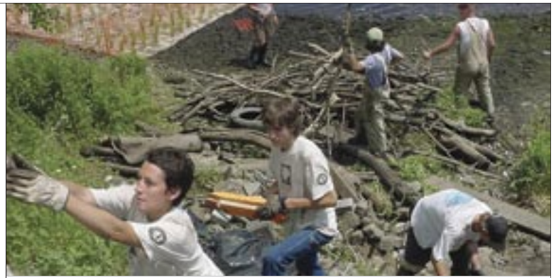
Salt marsh restoration work at the Concrete Plant on the Bronx River.
