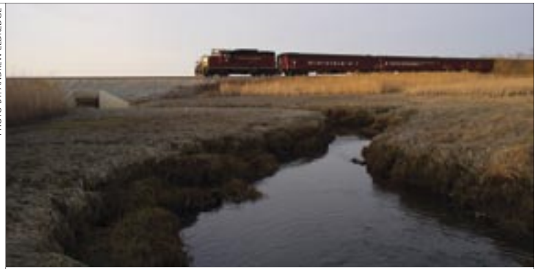
Train about to cross the newly-installed railroad culvert at Bridge Creek.
