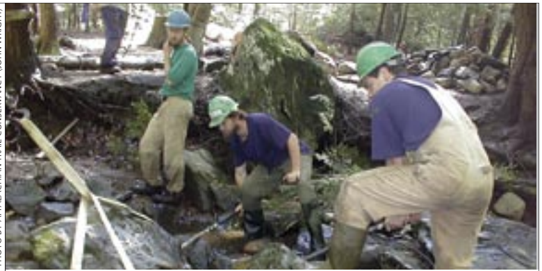
Volunteers and crew leaders of the Mid-Atlantic Trail Crew move stringers into place at Duell Hollow in New York.
