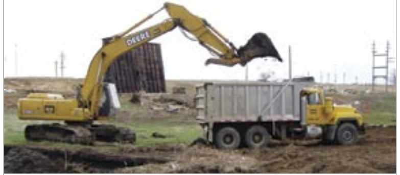
Cleanup of contaminated soil from a TNT manufacturing site.
