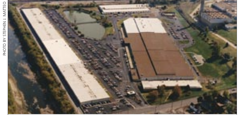
An aerial view of the National Imagery and Mapping Agency in St. Louis, Missouri.
