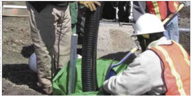
Workers planting trees in a deep hole for the phytoremediation project at Murdock, Nebraska - April 2005.
